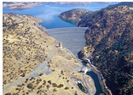
Virtual trades at CAISO’s New Melones intertie are at the center of market manipulation allegations filed by FERC in December. Source: U.S. Bureau of Reclamation
